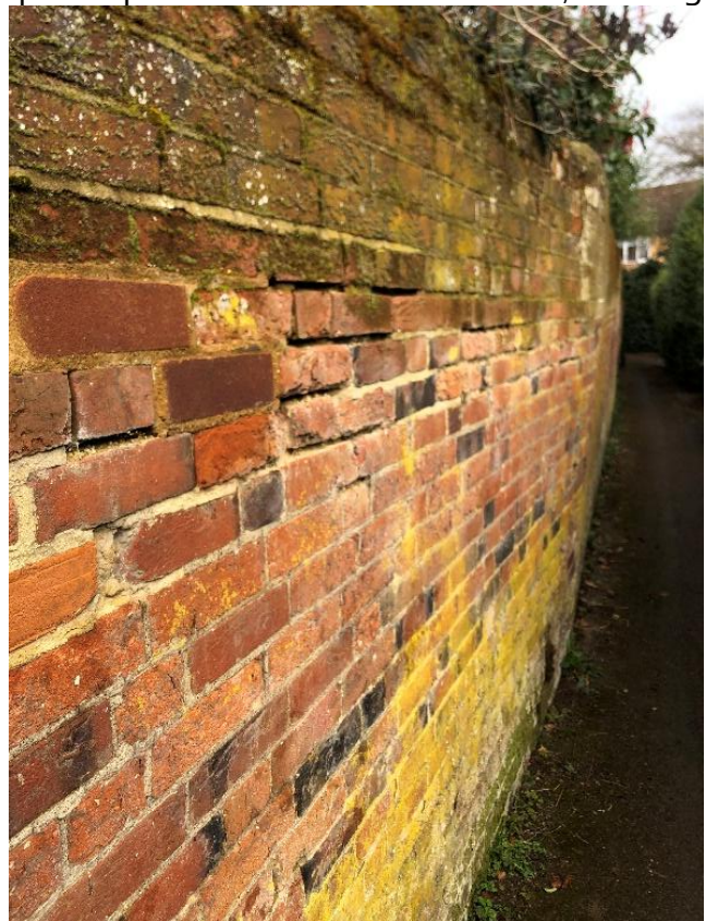
Another section of the wall which left to deteriorate will eventually collapse.
