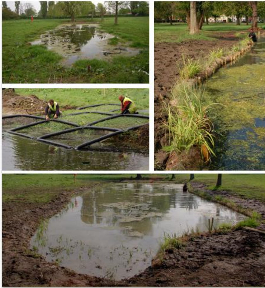
Above, clockwise from left: Pond before, Installing the bioroll, Pond after, Building the reed bed
