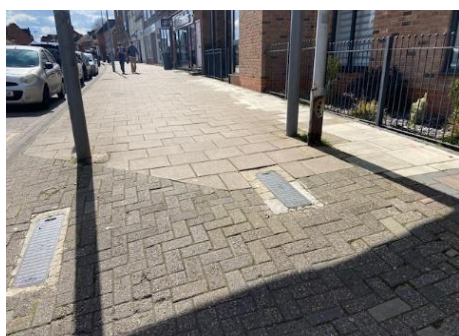
Cross-slope on vehicle access
