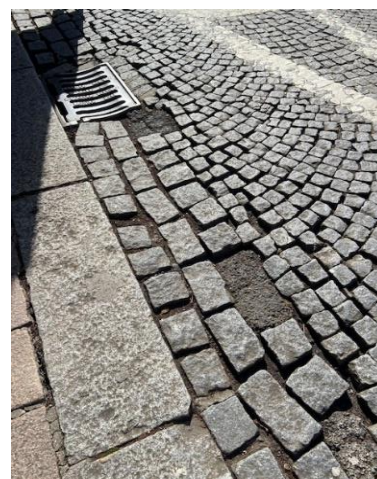
Loose or missing pavers
