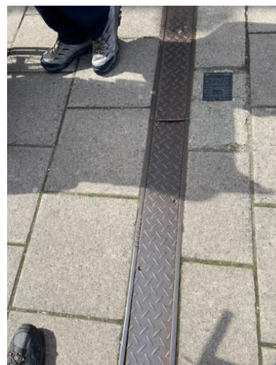
Steel / iron gully covers in poor repair
