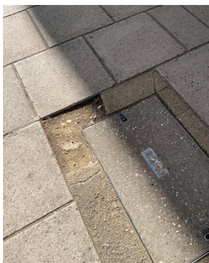
Damaged Concrete – frost damage or mechanical overload
