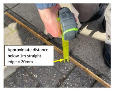
Paving stones are often uneven. It is easy to find examples of sections of paving where the deviation of the footway surface under a 1 metre straight edge is of the order of 20mm or even more (see picture left). This is well in excess of the recommended 3mm.
