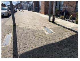
represents a major hazard. At present, the crossfall gradient is slightly shallower closer to the building, so Adrian tries to take advantage of this, having then to either pass between the fence and the signpost support and redundant (lamp?) post, or between the supports. There
