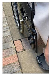
Generally the surface conditions are relatively smooth, but there is at least one dangerous gap between pavers where the mortar is missing. A few days before our survey, Sharon was nearly tipped out of the chair when the wheel became lodged in the gap (picture left) and Adrian suffered painful bruising.
