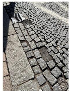
The cobbles in Market Square are a feature against which there is strong advice in the official guidance. As shown in the picture (left) they are poorly maintained making for a surface which is extremely uneven with many gaps large enough that the front wheels of a wheelchair can easily be caught between them. At the very least, they cause considerable potentially harmful vibration for both wheelchair occupant and carer.
