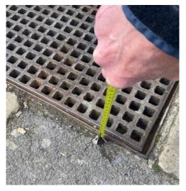
There are a number of inspection covers throughout this section of the route and not all are flush with the surrounding pavement. In the picture to the left, the surface of the grill is about 15-20mm above the surrounding tarmac and pavers. Steel grills and covers like the one shown can be slippery in wet conditions.
