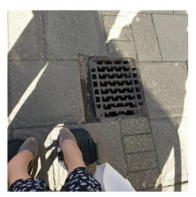
There are large gaps between pavers – sometimes of the order of 20mm or more in width and a similar depth – which should be filled with mortar. Where this is the case, sometimes the mortar is missing. Where this is in the direction of travel, it is possible for a wheel to be trapped in the resulting gap. When at right angles to the direction of travel, it contributes to steering difficulties and potentially harmful vibration for the wheelchair occupant.
