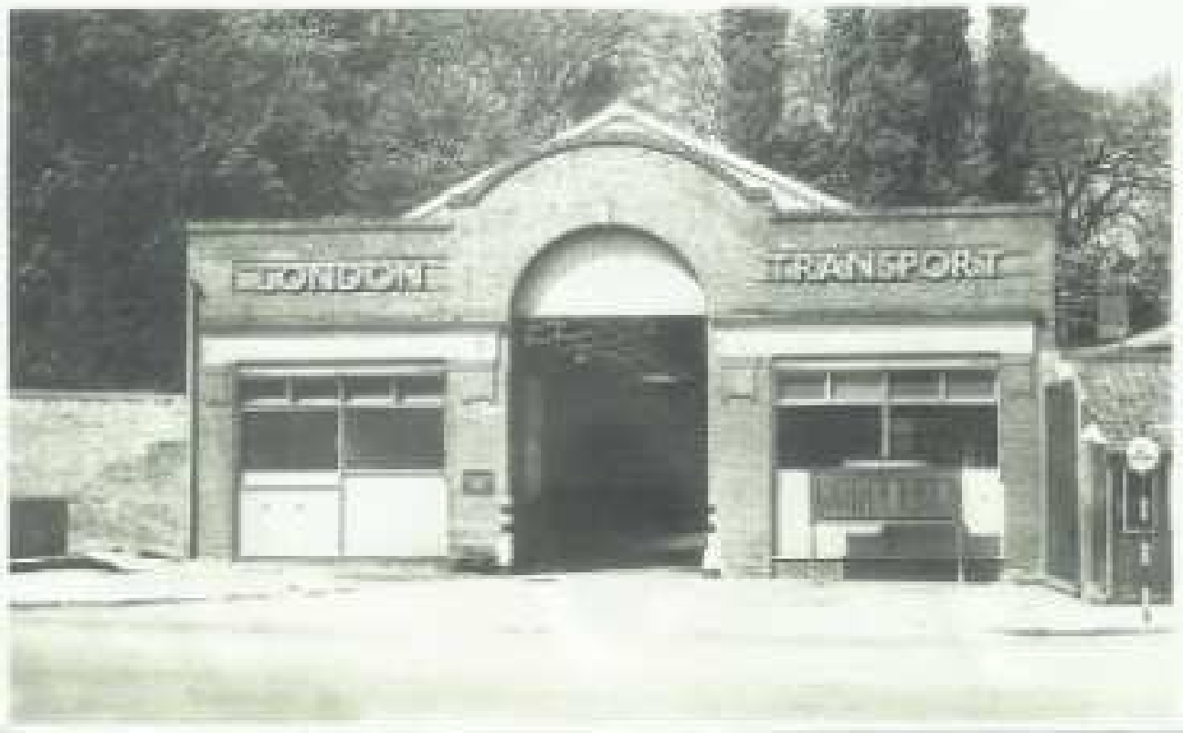
These two views of Hitchin garage show it as it was in 1928, with a new 10710 cubic yards and in 1935, after the busbores had been expanded to allow coaches to enter the depot. The alterations involved the removal of a portion of the existing walls so that the entrance doorway could be lifted to the level of the second floor of the old building and the installation of a higher roof, which can be seen rising above the old building in the 1935 view. The freight window has also been replaced by weatherboarding London Transport Motors.
