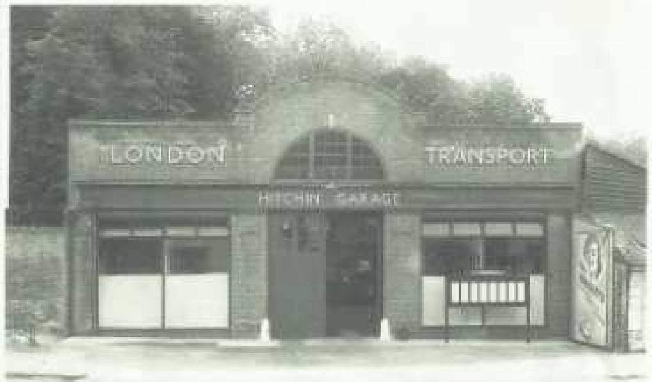
These two views of Hitchin garage show it as it was in 1928, with a new 10710 cubic yards and in 1935, after the busbores had been expanded to allow coaches to enter the depot. The alterations involved the removal of a portion of the existing walls so that the entrance doorway could be lifted to the level of the second floor of the old building and the installation of a higher roof, which can be seen rising above the old building in the 1935 view. The freight window has also been replaced by weatherboarding London Transport Motors.
